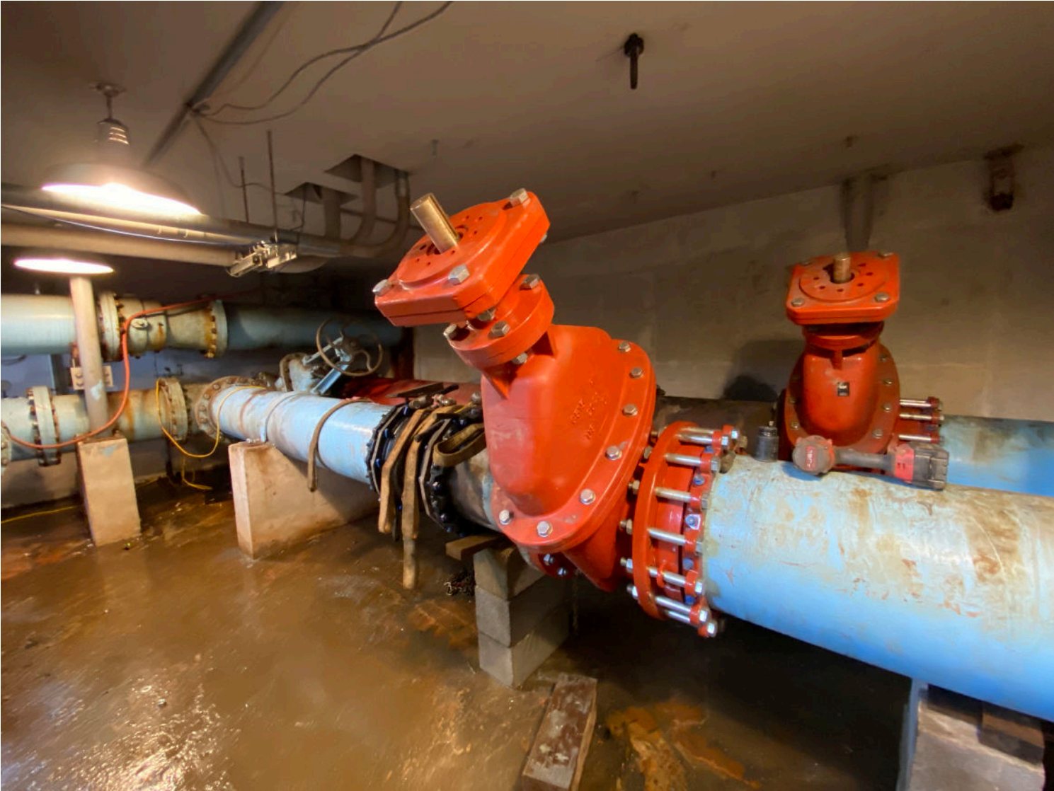
New Valves inside Booster Station No. 1
