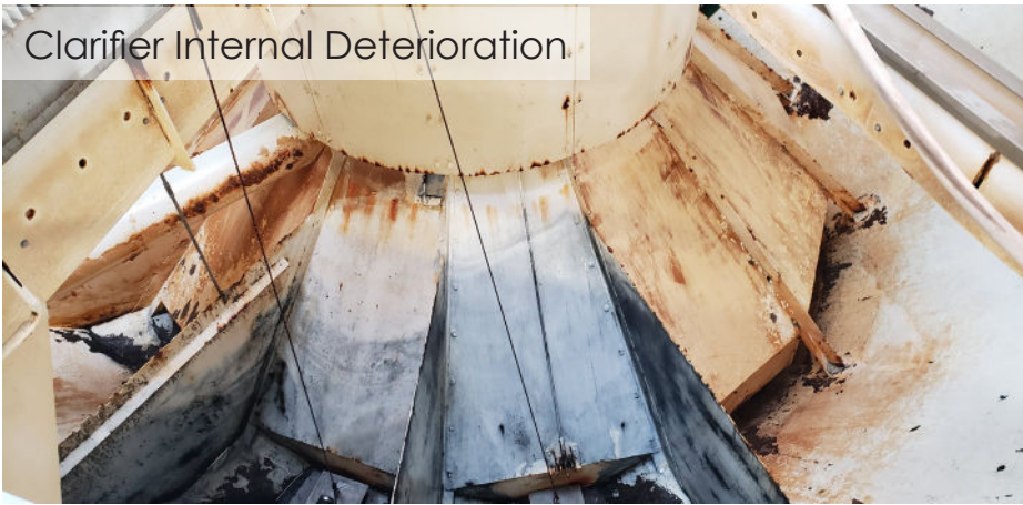
Clarifier Internal Deterioration
